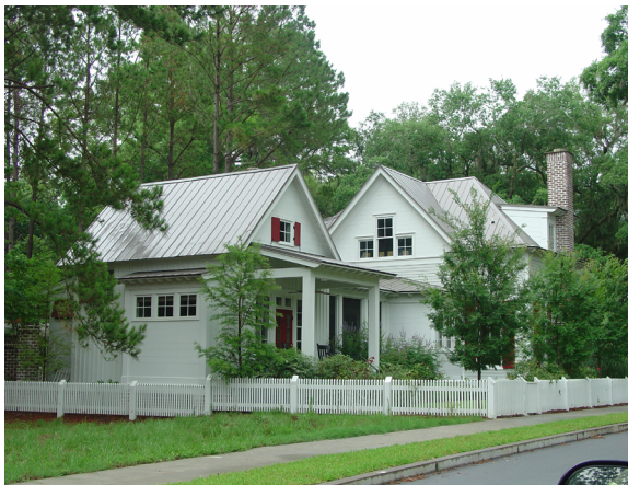
Demand for housing in the unincorporated County is mostly for single-family homes. However, accessory units like the one shown here offer affordable options in the more Rural Areas of the County.
